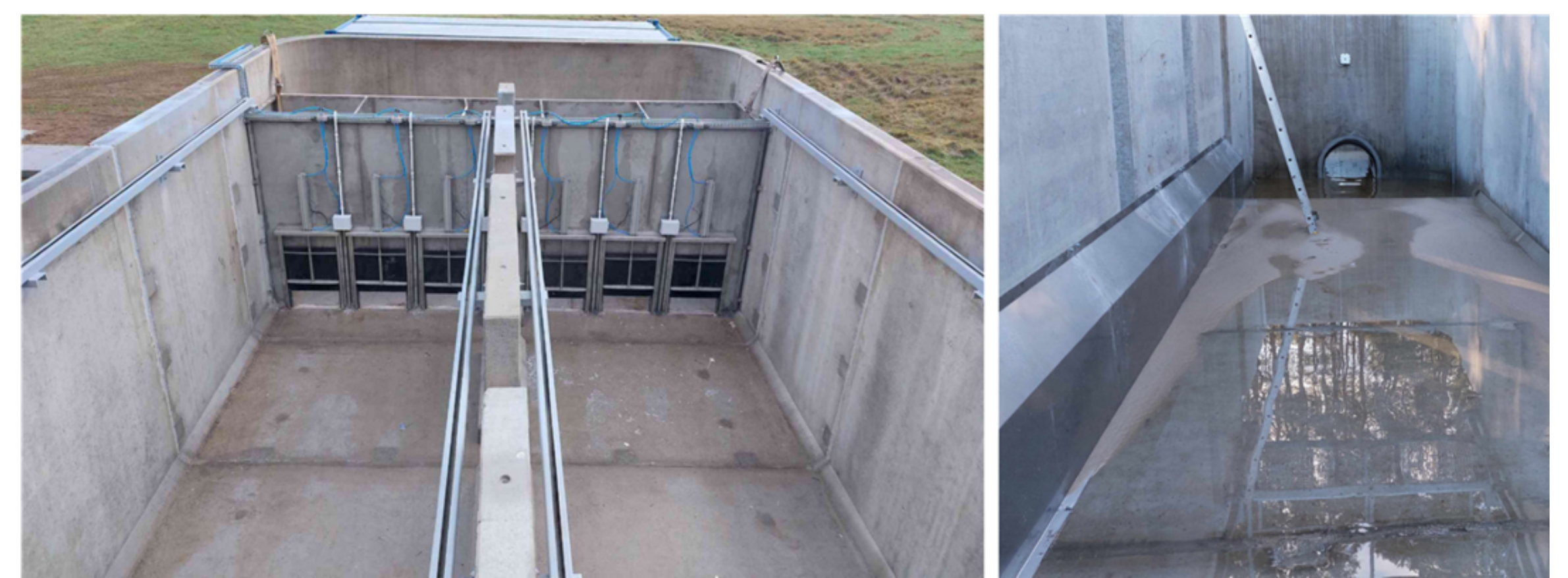
Figure 3: Flushing process at T = 2.4 m, a = 0.2 m, showing 100% substrate removal
